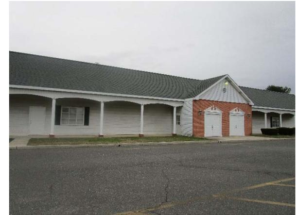
Parking spaces in the parking lot to the south of the building near the entrance can be converted to porous pavement to capture and infiltrate stormwater runoff from the parking lot. Two rain gardens can be installed at the back building's western entrance to capture and treat runoff from the roof. A preliminary soil assessment suggests that more soil testing would be required before determining the soil's suitability for green infrastructure.
